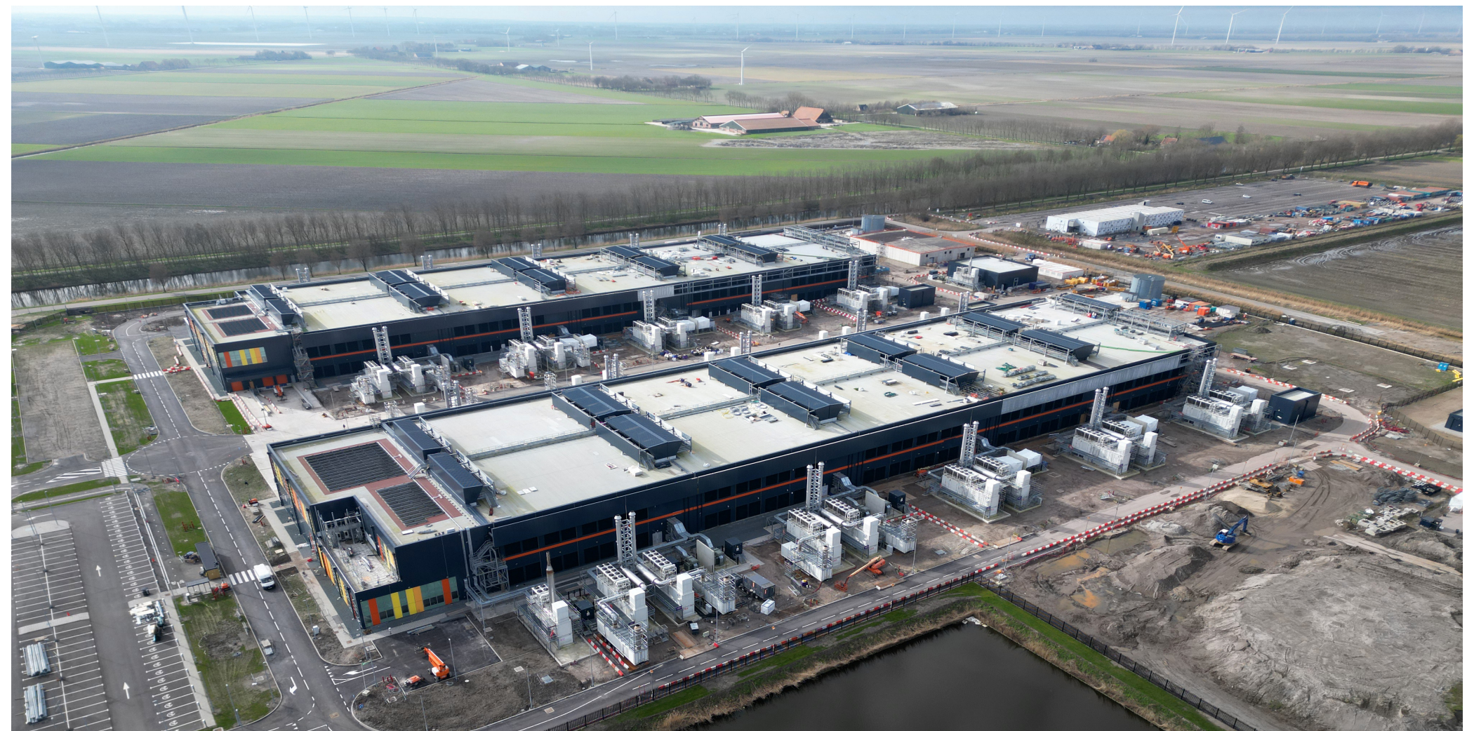
Figure1. Aerial view of a large datacenter in North Holland, The Netherlands By corlaffra (Adobe Stock)
